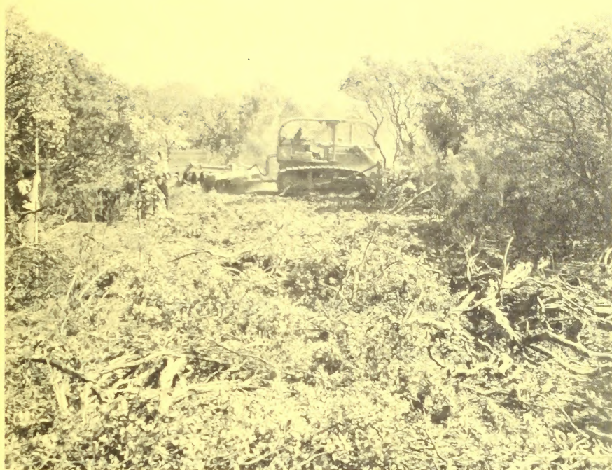
Fig. 13. Heavy duty disc can be used to crush large manzanita bushes. Manzanita here averages 15' high.
